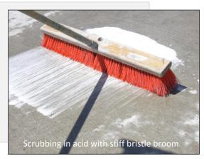
The acid should only have contact with the concrete for a maximum of 10 minutes. Triple rinse **thoroughly** with water (power washing is ideal) and allow to dry a **minimum** of 10-12 hours. Remove loose aggregate by blower, vacuum, or broom. In the end, your floor should have a texture similar to 80 grit (or rougher) sandpaper. Alternatively, Muriatic Acid can be used for additional profiling. (see website for tutorial)
