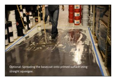
Once the material is out of the bucket and onto your substrate, it will take much longer for it to tack up (possibly up to an hour depending on surface temp and air temp). Higher temperatures will reduce the working life of the coating; lower temperatures will increase
