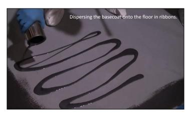
If you are using a roller to apply the Pure Metallic basecoat, you will need to roll fairly aggressively to move the material around. After the basecoat has been evenly dispersed, gently backroll the entire wet area with your roller (3/8" nap) in one direction to further promote even coverage.
